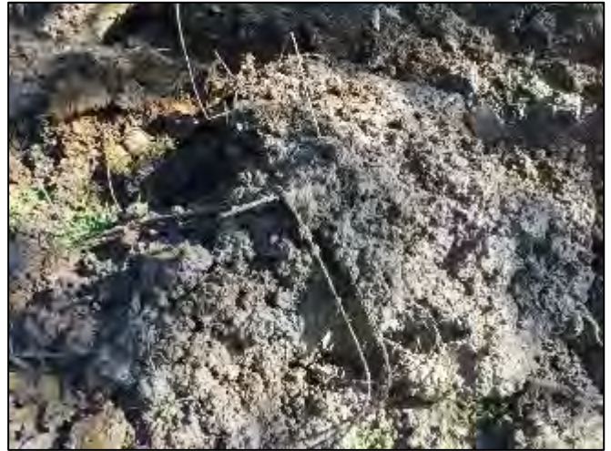
Plate 8 – Metal wire and fencing used as fill in the former dam.
