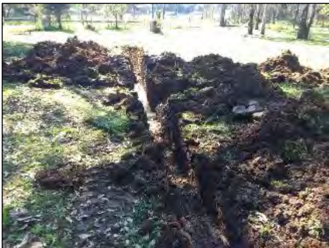
Plate 5 – Trenching across the former dam.
