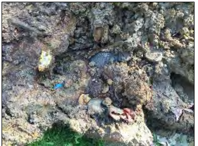
Plate 6 – Household waste used to fill the former dam.
