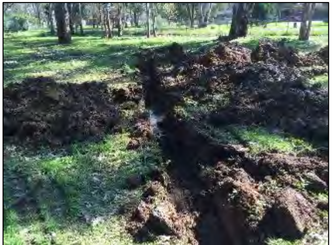
Plate 4 – Trenching across the former dam.
