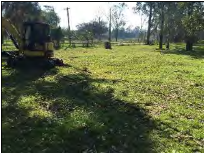
Plate 3 – Surface depressions in location of former dam
