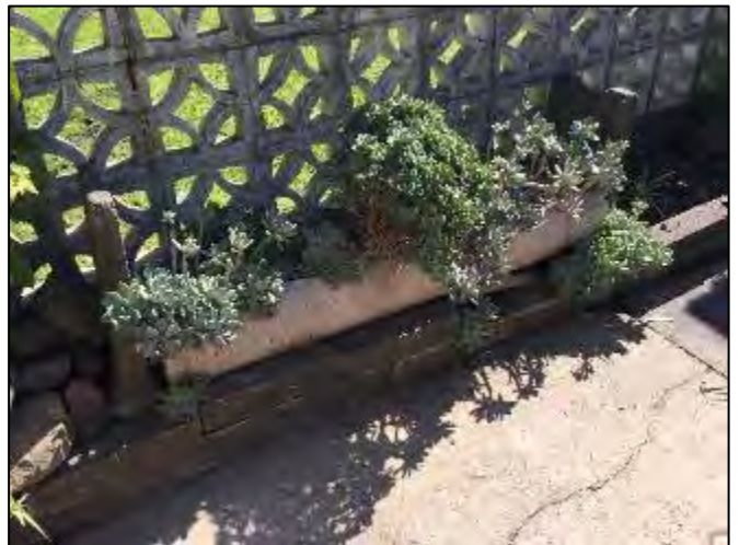
Plate 40 – Asbestos pipe used as planter box. Location of sample AC1.
