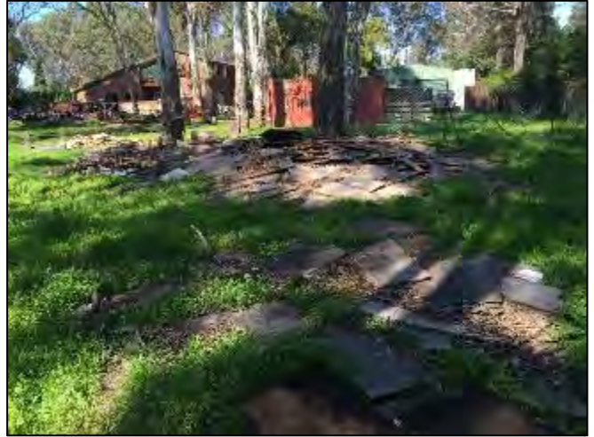
Plate 14 – Timber sheeting in the northern portion of the site. Note shipping container in background.
